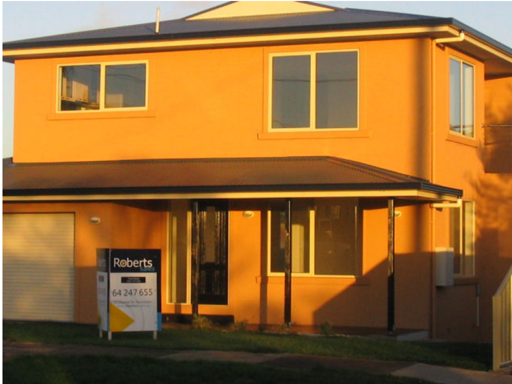
Texture Coating (Gunn Street Devonport Tas.)
